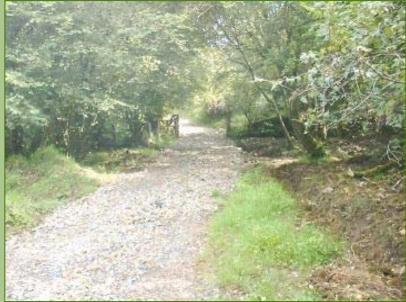
Improved track and stream crossing to minimise sediment inputs
