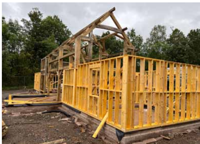
Use of Galloway-grown Sitka spruce in sustainable house construction in north Galloway. © John Paterson
